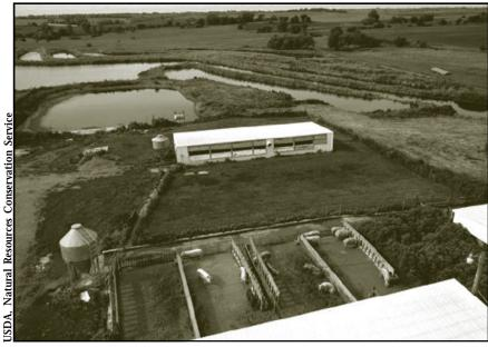
This hog operation in Taylor County, lowa, uses a wetland system constructed on a series of hillside terraces to filter and purify wastewater. Water quality tests indicated that the effluent from the treatment wetland was cleaner than that required for wastewater treatment plants.
